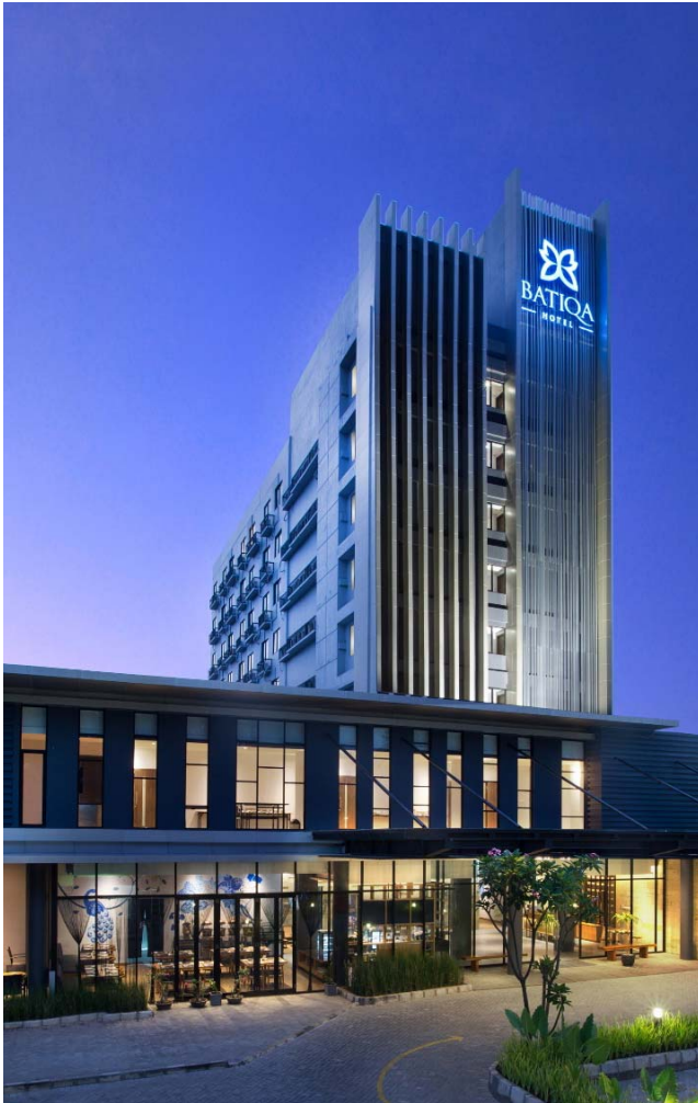
Exterior view of BATIQA Hotel Cirebon
